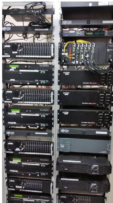
Typical Voted-Simulcast Head End Radio Site – showing an Orolia SecureSync, five voters, and other radio accessories.
