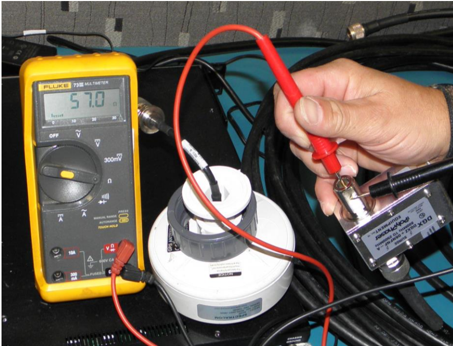
Figure 22: Checking the impedance of an antenna through the “GPS suppressor”
